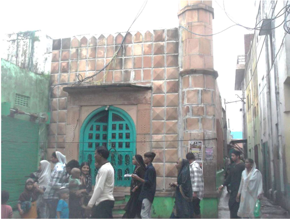
Image 17: View of approach to religious precinct- “Hatai Masjid” with narrow lanes towards South in the Regulated Area.
