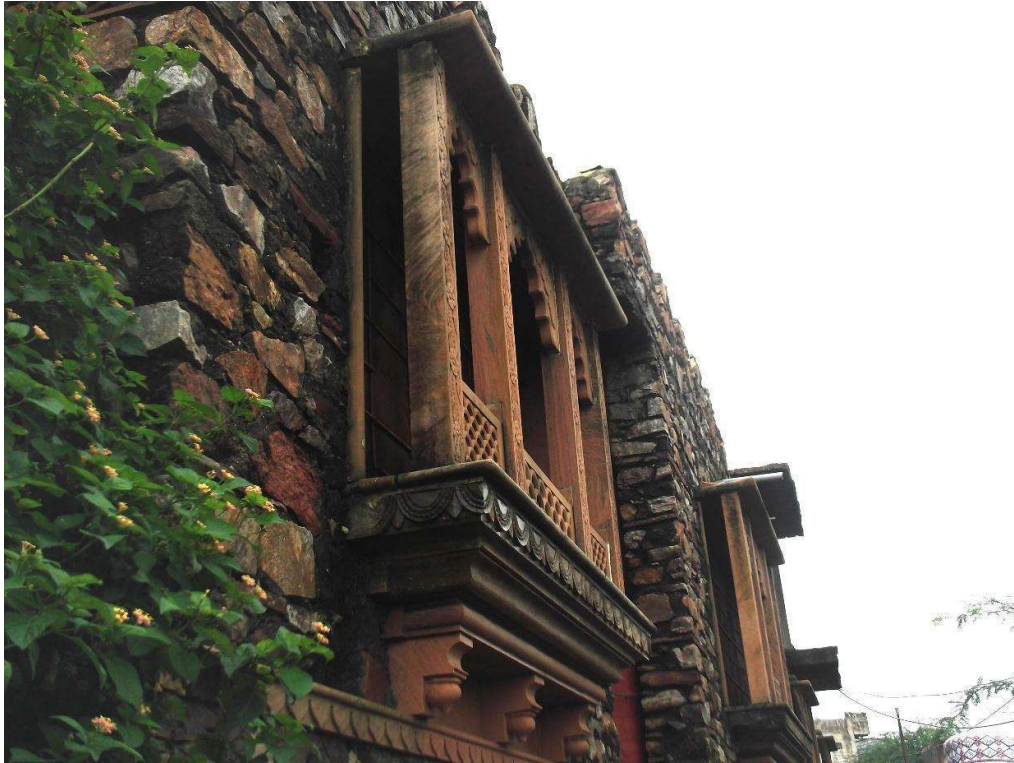
Image 13: Architectural Elements showcasing Rajput Architectural style in ‘Taragarh Fort Wall’ towards the North East in the Regulated Area.
