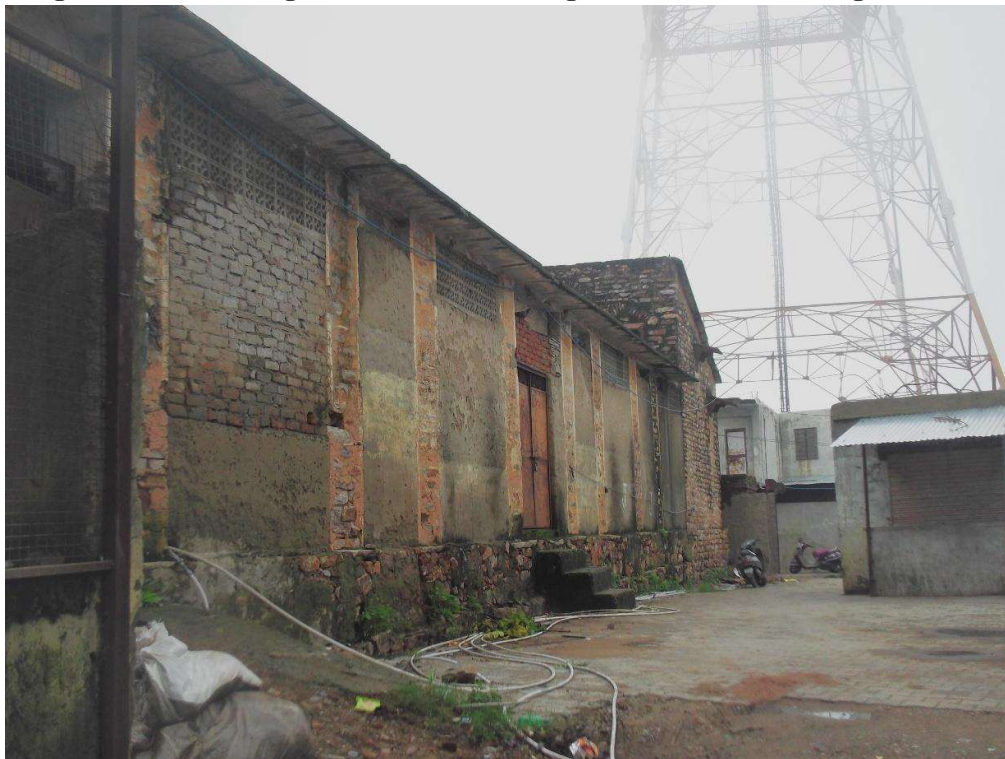
Image 16: View of abandoned stone structures with view of Taragarh Tower at the backdrop towards the East in the Regulated Area.
