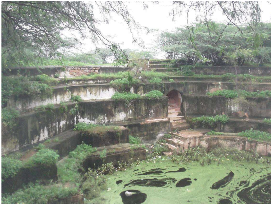
Image 12: View of octagonal water body ( bawdi ) towards the North East in the Regulated Area.
