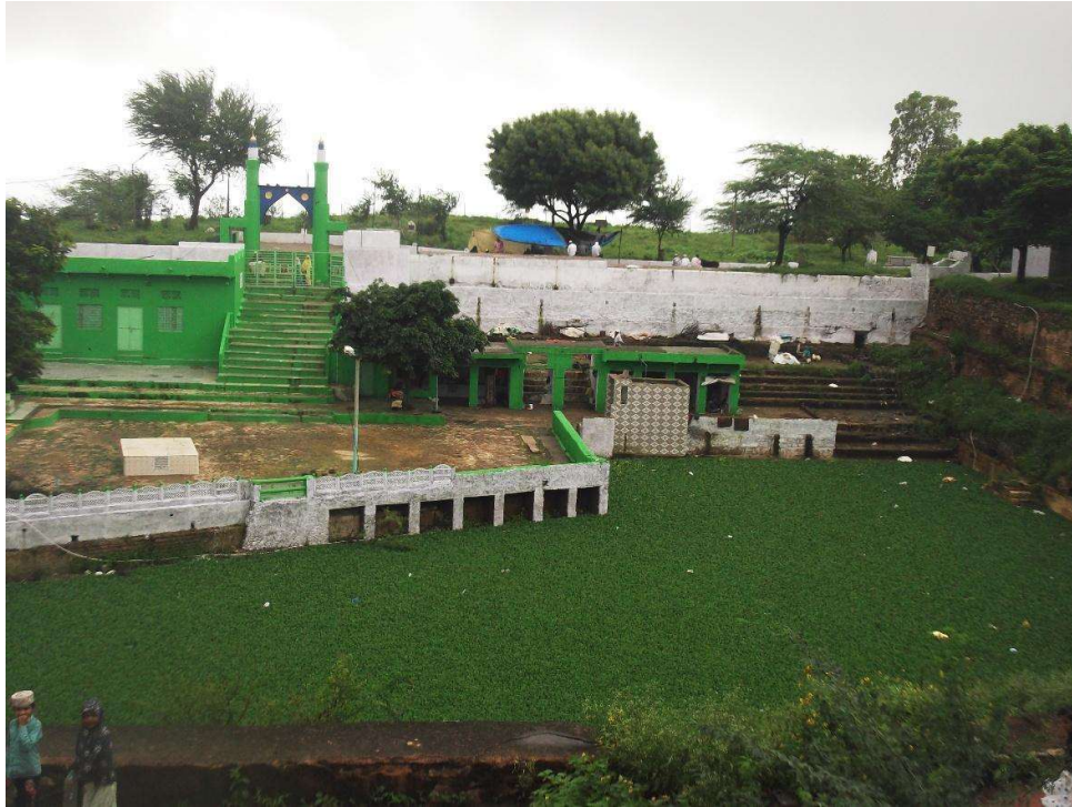
Image 21: View of pond locally known as jhalara inside the complex of ‘Roza-e-Imam Hussain RA’ Mosque towards the South East in the Regulated Area.
